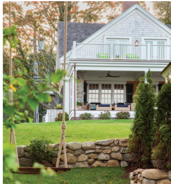
The steep slope to the harbor (top) provided Ahearn with the opportunity to create a garage and utility structure without interfering with the marvelous water view.
