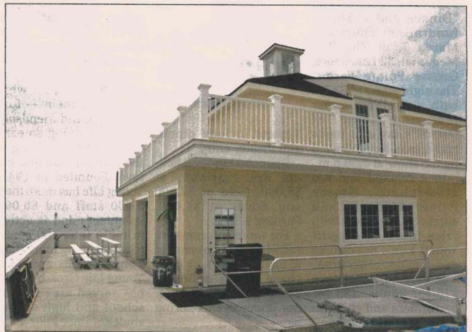
The Marine Activity Center was added to the club in August 2017.
